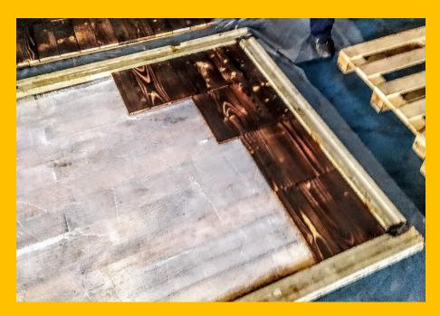
After positioning the boards and applying the first layer of resin, the fiberglass is laid down, followed by the second layer of resin and pallet boards. Then, the panels are charred using the Shou Sugi Ban technique, brushed, and coated with boiled linseed oil. The walls are now ready for installation: the first horsebox made from reclaimed materials.
